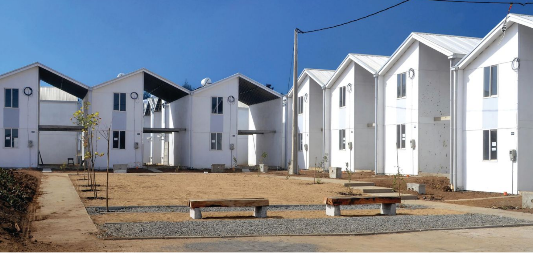
VILLA VERDE HOUSING, 2013, CONSTITUCIÓN, CHILE., PHOTOS BY ELEMENTAL TOP: "HALF OF A GOOD HOUSE" DEVELOPMENT, FINANCED WITH PUBLIC MONEY. BOTTOM: MIDDLE-CLASS STANDARD ACHIEVED BY THE RESIDENTS THEMSELVES.
