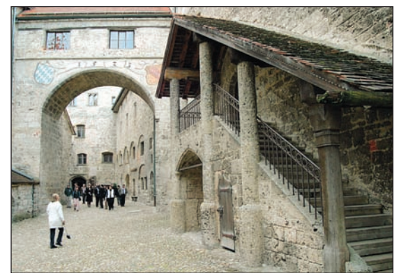
A staircase leads to a second-story floor inside Burghausen Castle. Above the archway is the year 1523, but the oldest parts of the castle date to 1255.
