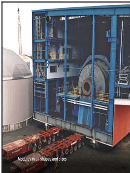
Figure 2 Red Dog Mine Modular Build, began operations in 1989, Courtesy of Mammoet. Note the two Self-Propelled Modular Transporters (SPMTs) carrying a large module containing what appears to be a Fuller 22 foot diameter by 8.5 foot 1500 kw, 2000 hp SAG Mill and ATCO offices. Photo Courtesy of Mammoet.
