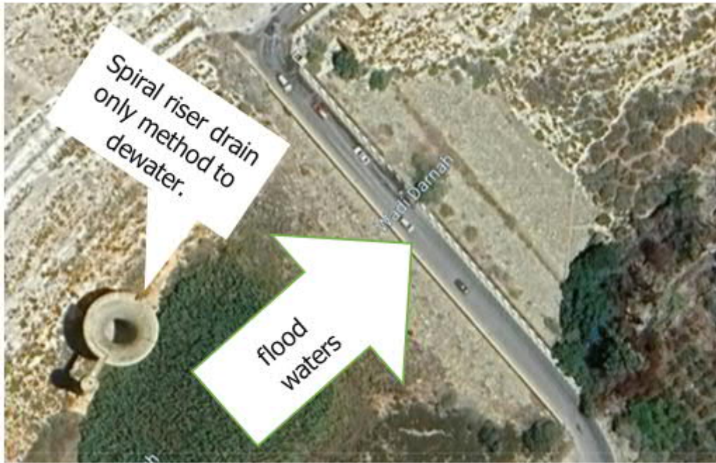
Figure 3 Abu Mansour Dam, downstream of the Al-Bilad Dam failed September 10. Dam had a spiral riser pipe, with no emergency spillway. Author's figure. Source: Google Earth
