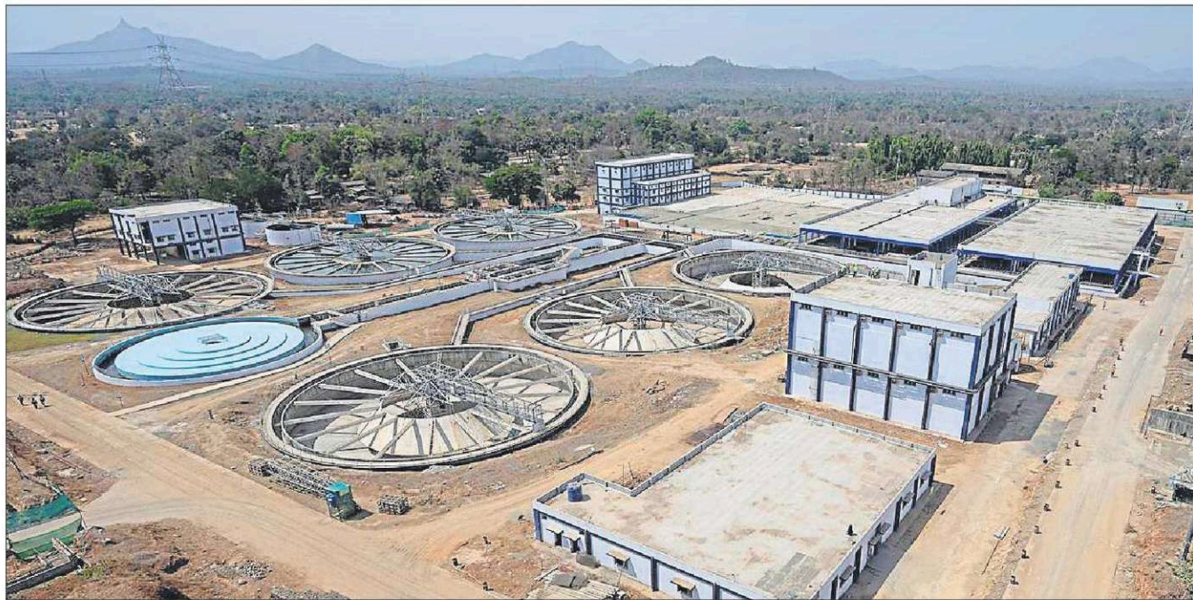
The water treatment plant, in Dahanu, is recognisable by six circular reactor clarifiers.
