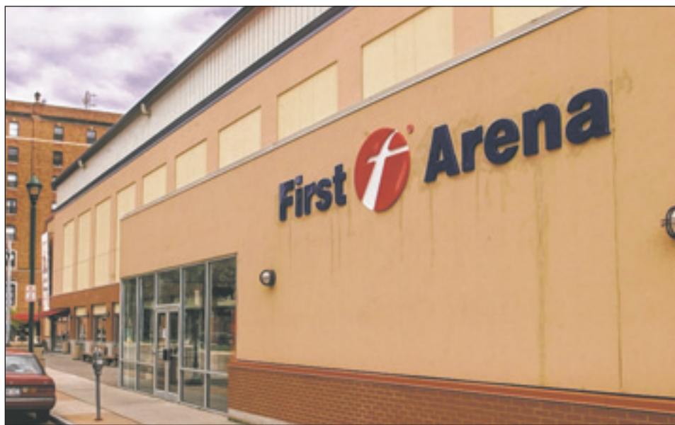
Problems with some sprinkler heads were found by inspectors as far back as 2005 and 2007, according to records obtained by this newspaper. County Executive Tom Santulli said he has been concerned about the arena's safety since it was seized in foreclosure. FILE PHOTO
