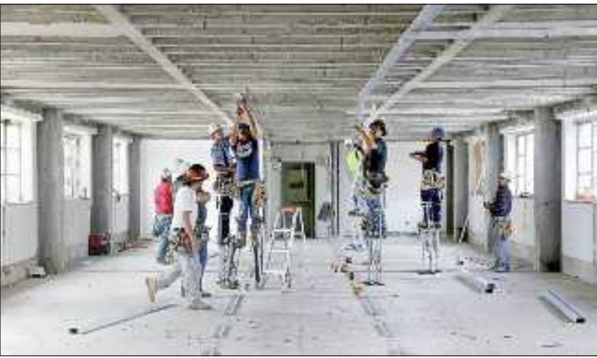
Workers install metal studs that will become the walls of the individual apartments on the fourth floor of the downtown YMCA building Friday. The demolition phase is nearly completed and construction has begun on some floors.
