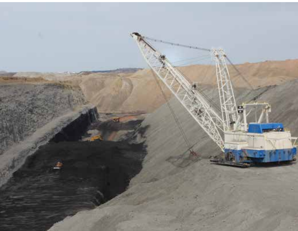
The 9,000-acre Spring Creek Mine produces an average of 50,000 tons of coal each day from its 80-foot-thick coal seam. Here, a dragline moves overburden away from the coal. Each bucketful holds nearly 80 cubic yards of material, more than 100 tons. PHOTO BY JOSEPH T. O’CONNOR
