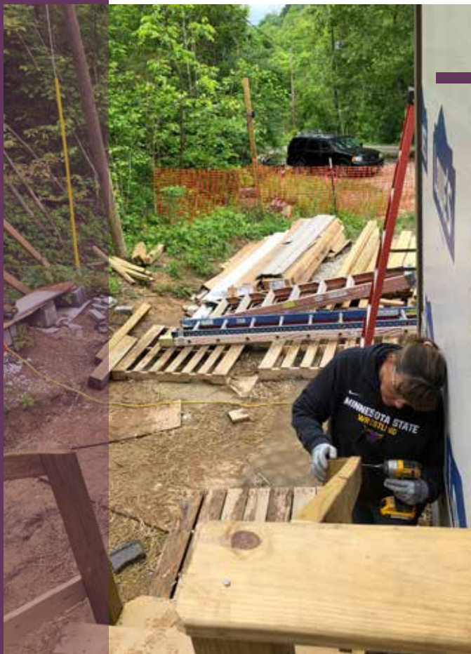
Bernadette Beckman works on building the back porch.
