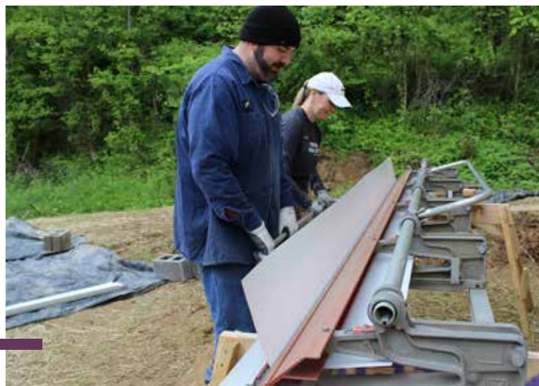
(l-r) Barker and Musser work together on bending fascia.
