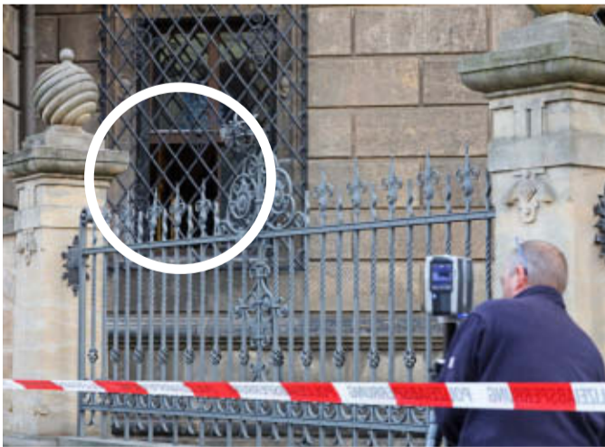
Entry point: The wrought-iron grille, circled, in a ground-floor window through which the tiny thieves squeezed into the building
